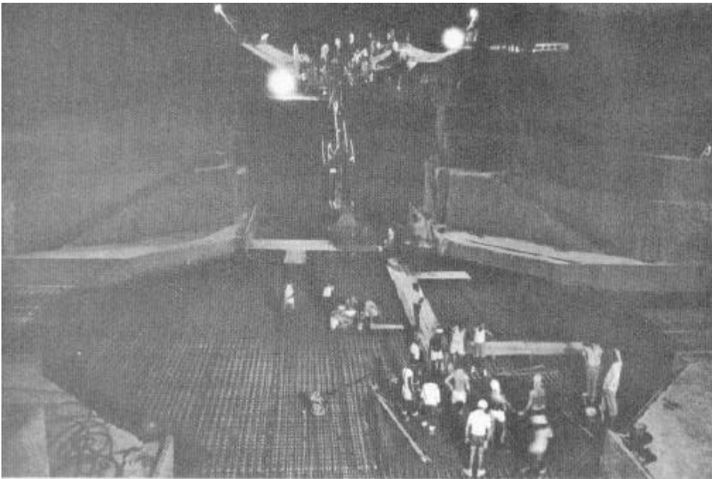
Concreting went on day and night for 26 hours
