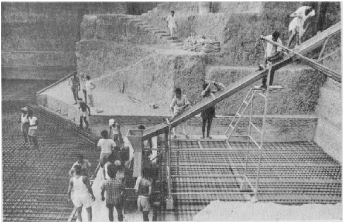
Starting to pour the concrete of the 22cm thick tie-slab
